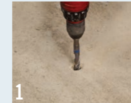
1 Use a 16mm drill bit to ensure the correct depth for the plug.
