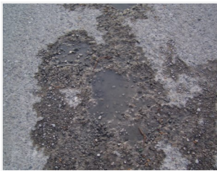
Rain / Frost Damage - Page 5
