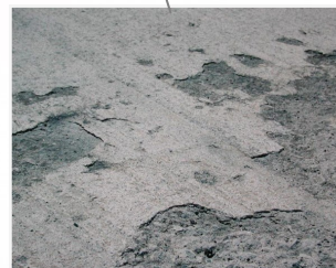
Scaling & Shallow Defects - Page 8
