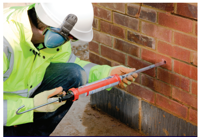
Injecting resin to complete the RetroTie installation
