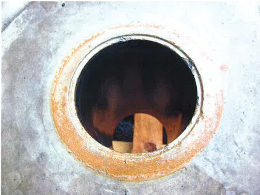
Figure 5: View - top of the test setup; concreted-in coated liner pipe ZVR DN 100
