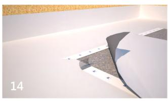
To complete the overlapped joints, peel off the protective release liner from the adhesive edge of the HydroBond Tape and press the laps together. Use a hard roller to ensure the laps are fully and constantly adhered.
