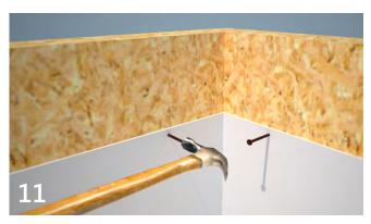
Nail the membrane to the formwork leaving the nails exposed to give a key for the concrete and to ensure that the formwork can be easily removed. The nails are cut flush with the membrane after the formwork is removed. A dab of 106 FlexProof or 109-LM can be used over the small hole, although the membrane will self-heal.
