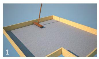
Sweep the support surface clean. Substrate should be smooth and firm. Concrete surfaces should be free of voids and sharp projections. Surface irregularities should be removed before installation. Voids must be filled with mortar, and holes filled with proprietary non-shrink mortar/grout.
