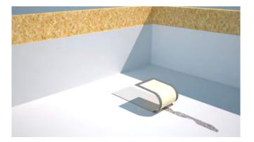
HydroBond Tape, pressing firmly using a hard roller to ensure a good bond. Overseal the outer edge of the patch with Newton Mesh Tape. Use a hard roller and a heat gun to fully adhere the Mesh Tape into the membrane fleece.
