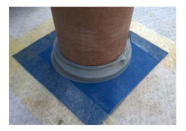
This can be tested to DIN 1048/BS EN 1542 and the level of full bond and suitability of use is relevant to both the water depth/pressure tested for both lateral migration and watertightness of the membrane and the laps.
